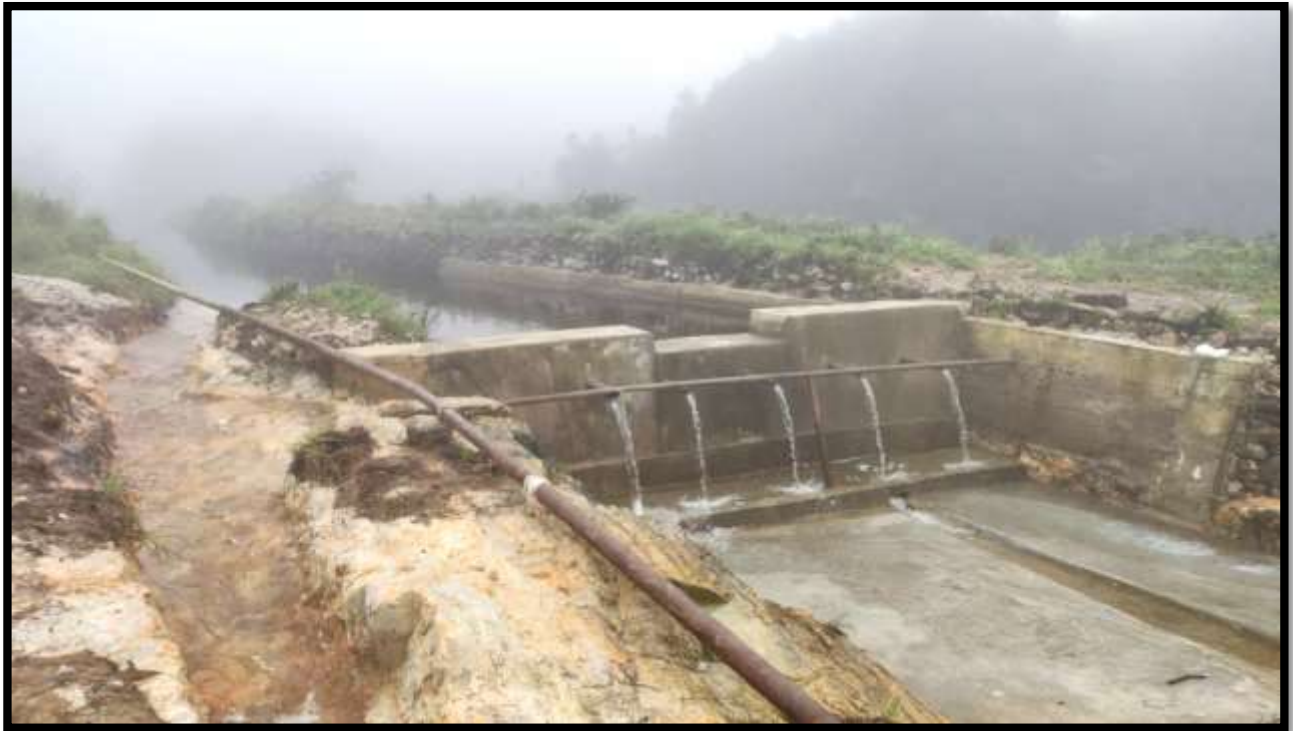
CHECK DAM AT LYNHING (UPPER UMJAR WATERSHED)
